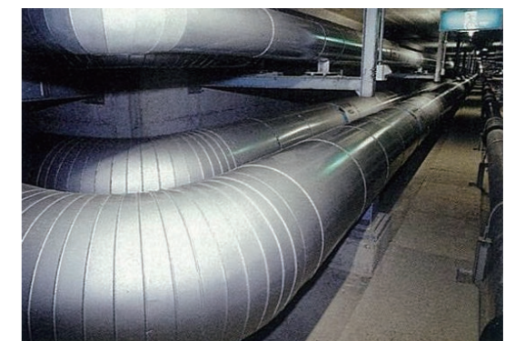
Pipeline (in public conduit)
