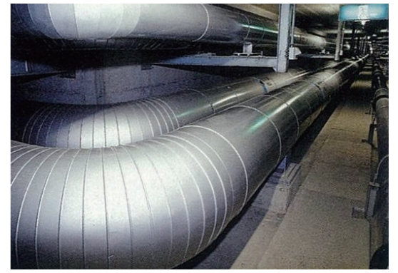
Pipeline (in public conduit)
