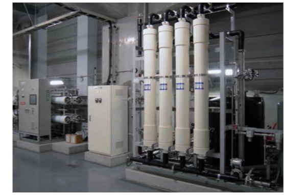
Water-saving cooling water recycling equipment
