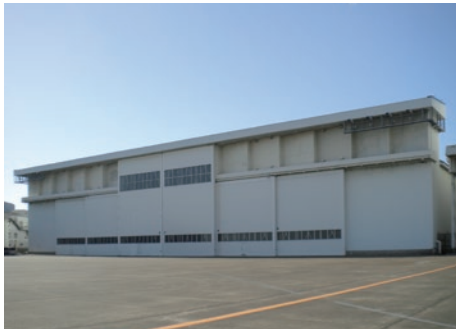
Large-scale hangar (near Runway B of the former aircraft maintenance area in Tokyo International Airport)
