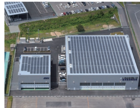
Solar panel on the rooftop of hangar in Kagoshima Airport
