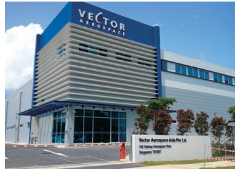
Engine maintenance plant (Singapore Seletar Airport)
