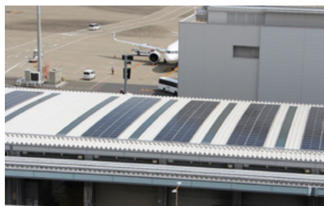
A solar power generation facility for inhouse use in Haneda Airport domestic cargo terminal (left) A hybrid freestanding light (right)
