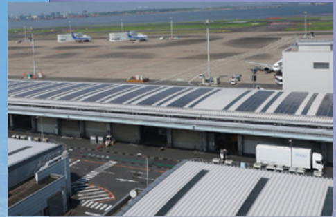
Solar light power generation (rooftops of the domestic cargo terminal of Haneda Airport)
