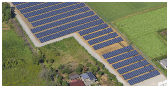
Solar power generation facility utilizing the idle land (Honsanrizuka)
