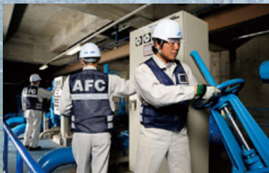
Inspection of water supply and drainage facilities
