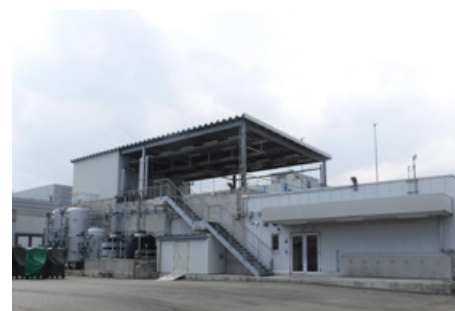
Large-sized aircraft washing facility
