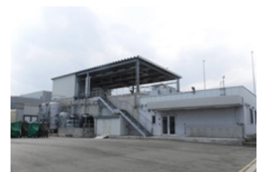
Large-sized aircraft washing facility
