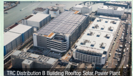
TRC Distribution B Building Rooftop Solar Power Plant
