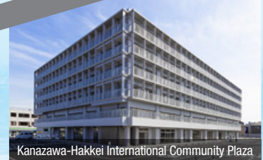
Kanazawa-Hakkei International Community Plaza
