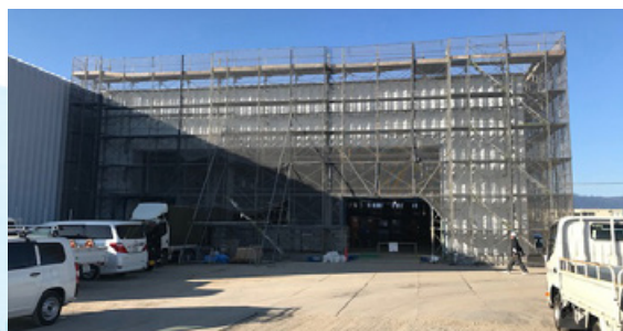
Extension work of Kobe Hangar
