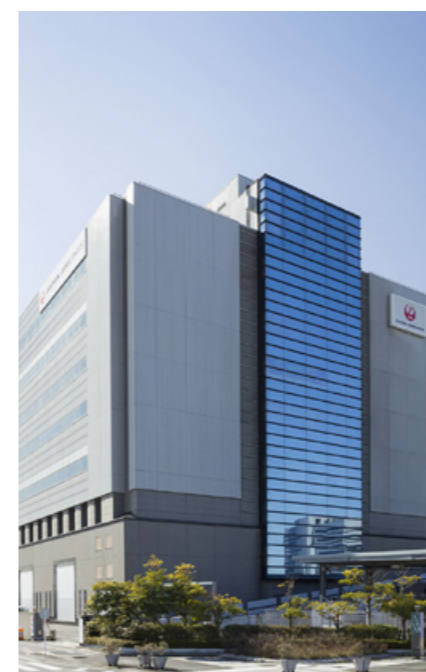
Technical Center 1 (Haneda Airport)
