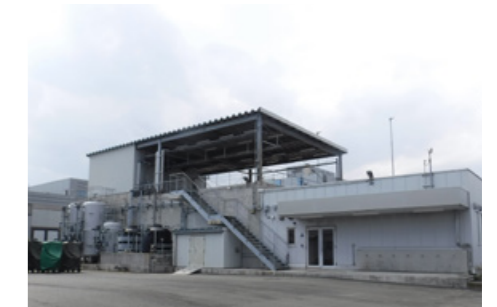
Large-sized aircraft washing facility
