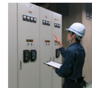
Maintenance and inspection
