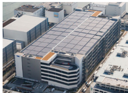
TRC Distribution B Building Rooftop Solar Power Plant
