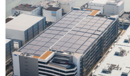
Solar light power generation (TRC)
