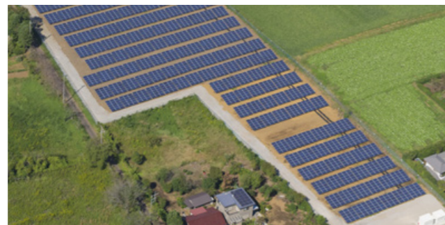
Solar power generation facility utilizing the idle land (Honsanrizuka)
