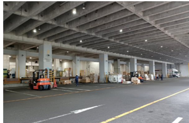
Rinku International Logistics Center
