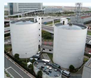
給排水施設 Water Supply and Drainage Facilities
