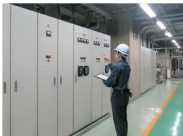
点検業務 Inspection work
