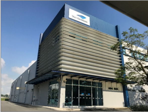
[Engine maintenance facility]
