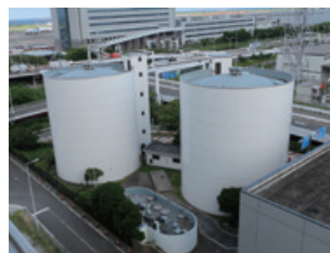
Water supply & drainage facilities in the reclaimed land area offshore
