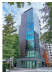
Nihonbashi-Hamacho 2-Chome Building
