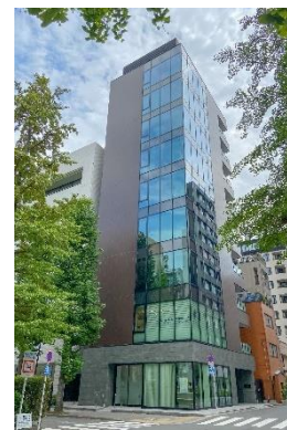
Nihonbashi Hamacho 2-Chome Building
